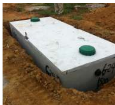
COMMON SEPTIC TANK
