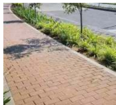
WIDE RCC ROAD BOTH SIDE PAVING
